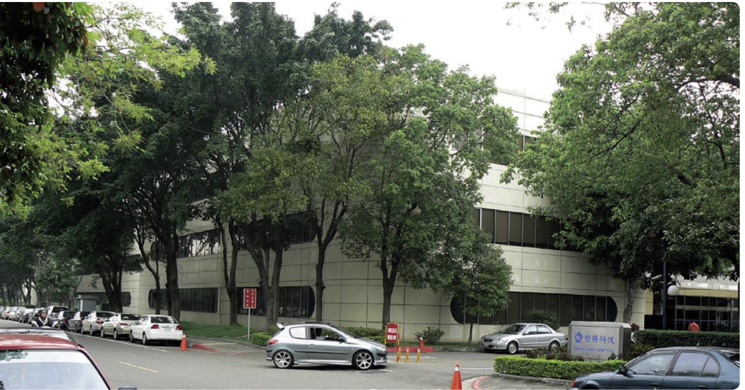
The Hsinchu Science Park in Taiwan carries the name “park” appropriately: hidden behind the trees are the offices and production facilities for MTI.
