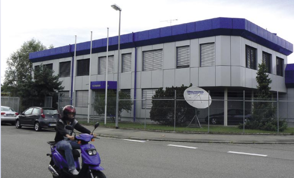
■ A look at the office building of company Spaun in Singen in southwestern Germany. Behind the building to the right can be found the production facilities for Spaun's multi-switches.
