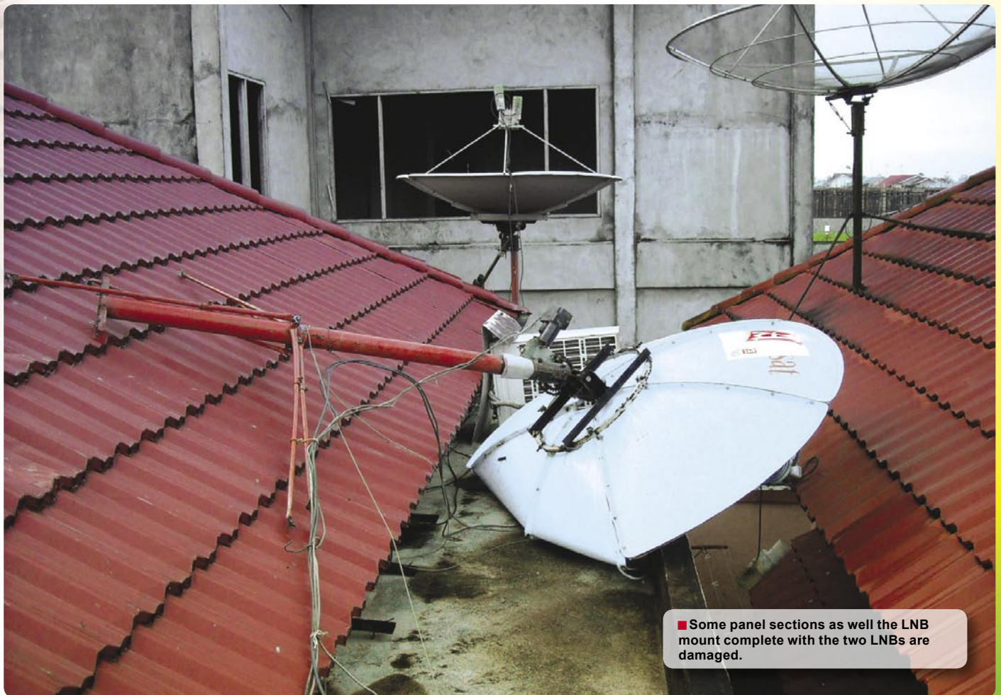
■ After: What a shame – the 1.8 m dish has collapsed due to high wind loads.
