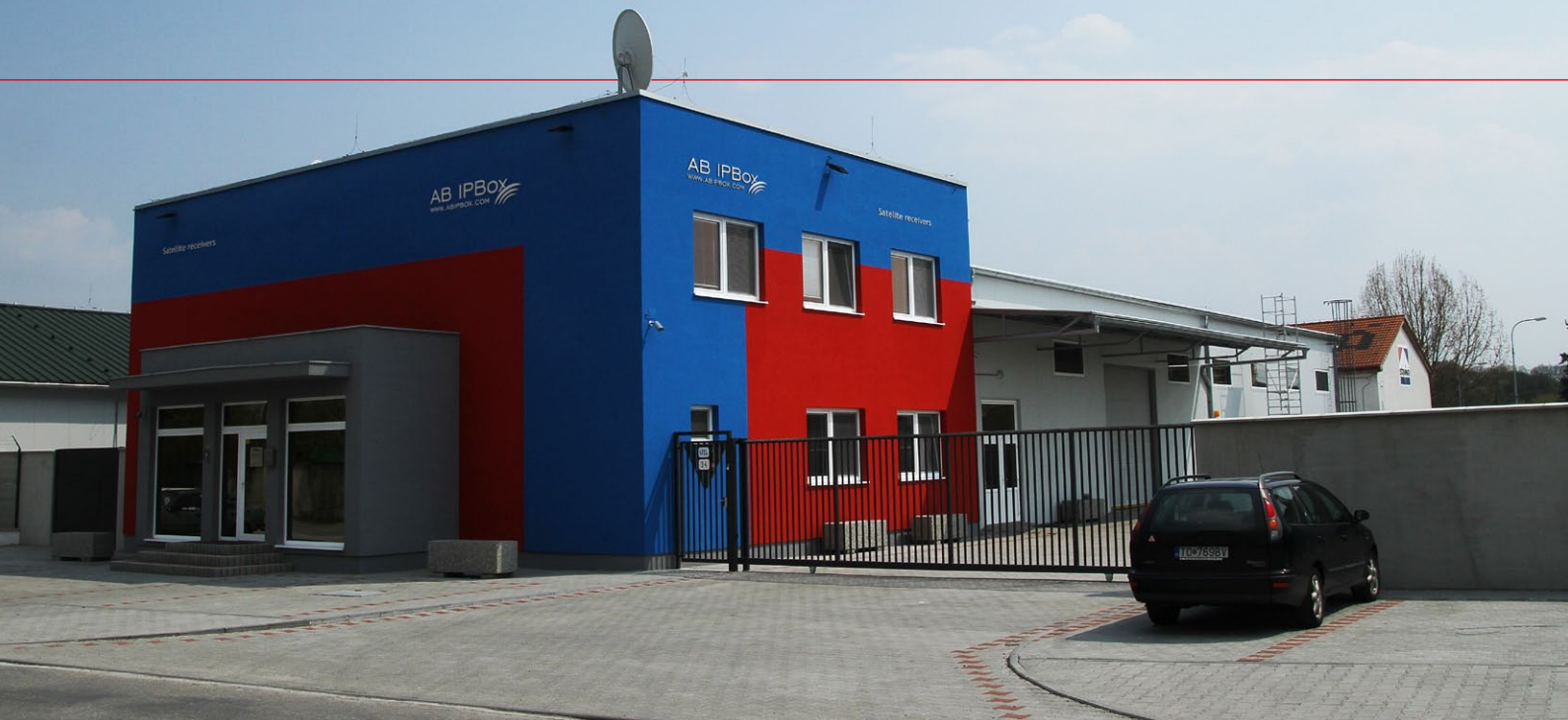
■ ... and again in 2010. The two-storey administrative building can be seen in front, with warehouse and dispatch and repair facilities in the back.
