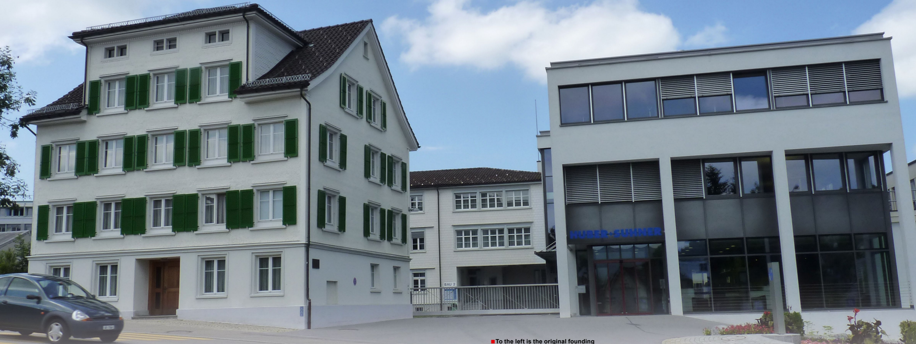
■ To the left is the original founding building of the company SUHNER back in 1869. To the right is the new reception building of the merged worldwide company HUBER+SUHNER.
