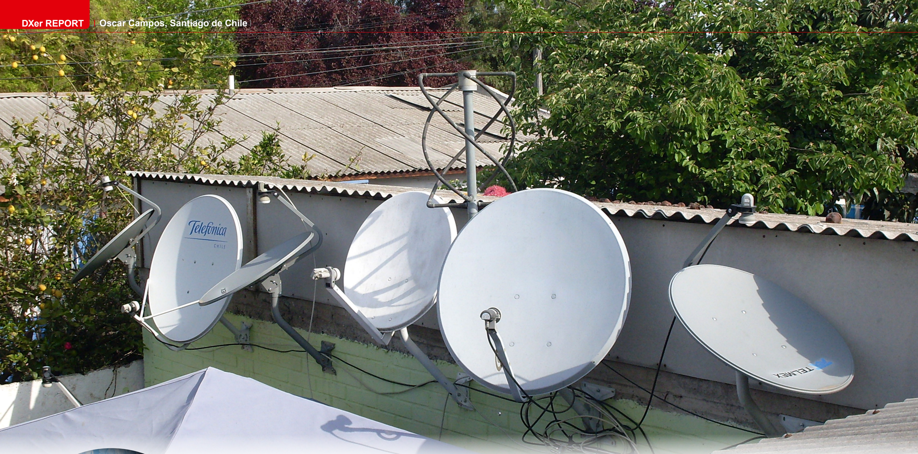
■ Oscar Campos mounted six 70cm dishes in a row: three of them were installed normally while the other three were installed in the inverted position. In the middle is a Helix antenna for the reception of the NOAA weather satellites.
