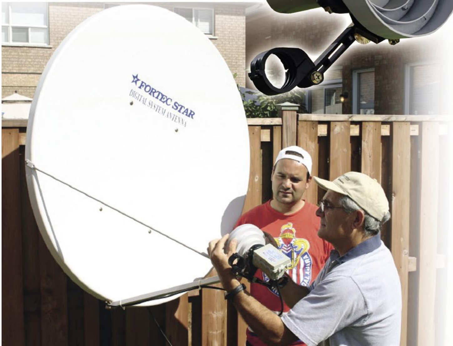
| Scalar Ring Cone-shaped | Vito dan Tony Memasang Antena 1,2-Meter
