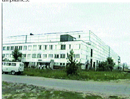
The front view of SUPRAL building
