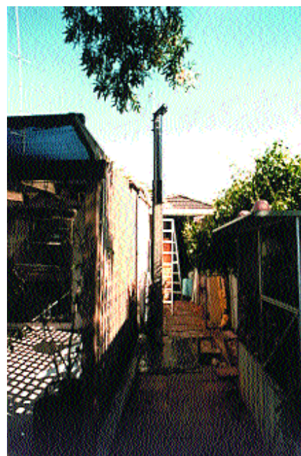
This shows the strings on the side of the tower with the centre pole extended about a metre. When the dish is mounted this pole telescopes out the top of the tower 2 metres. The pole retracts for servicing as well.
