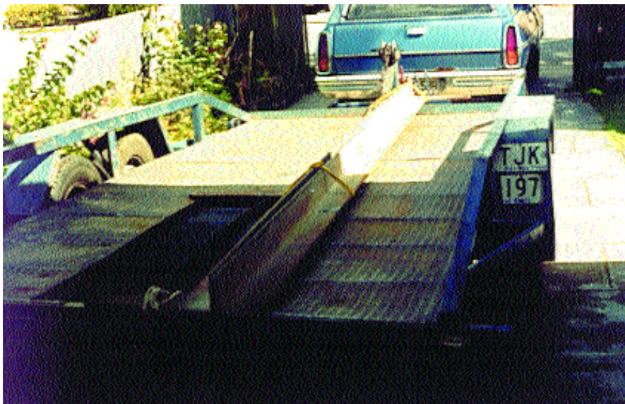
The two pieces of angle iron on the trailer. The two extensions on the end were used to hang the insulators. They are now 6 feet under and helping to resist any twist that may occur.
