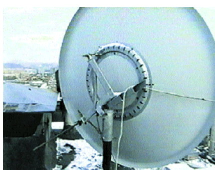
Polarmount of 1.65m SUPRAL dish
